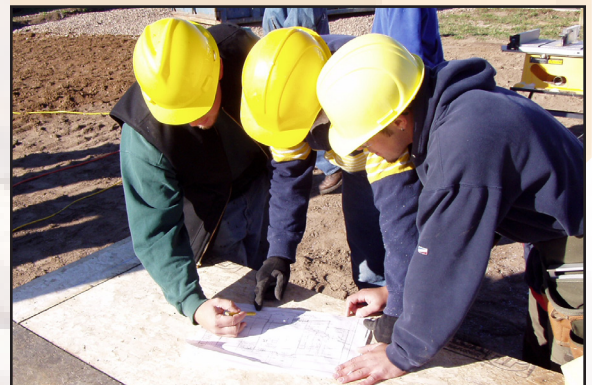
Students apply construction print reading skills in the field.
